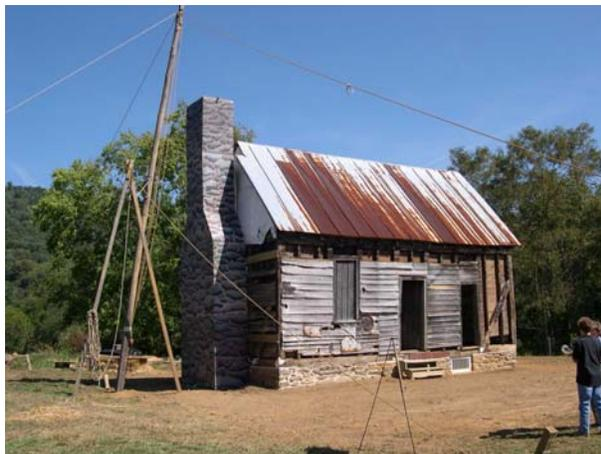
The Hollow in October 2005. Note the perfectly restored foundation. The chimney is a temporary wood and paper replica for the JM house tour.
