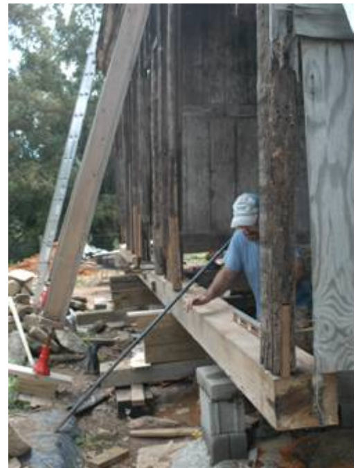
Ahead of the photographer's arrival, Mike had nearly single-handedly completed strapping and lifting the south oak sill into its receiving vertical and horizontal tenons. However, he good-naturedly accommodated documentation of the significant event by gently loosening a few still unfastened joints and straps for partial re-creation. Proving more stubborn this time, Edward joined the effort to lift and push the sill into receiving tenons. Note to their credit, the sill is perfectly level and the tenons are fully in place in the two bottom pictures, 8/31/2005.
