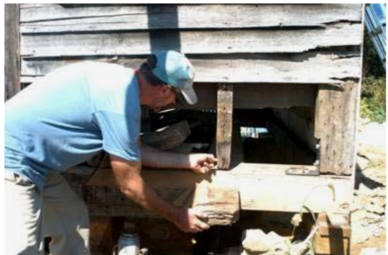
Mike demonstrates where he found the hollowed-out sill in alignment with his positioning of the hearth girt, visible in the shadow behind the stud he points to.
